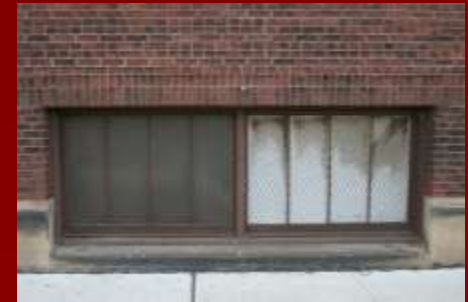
HOPPER/AWNING WINDOWS (PROJECT IN & PROJECT OUT)
