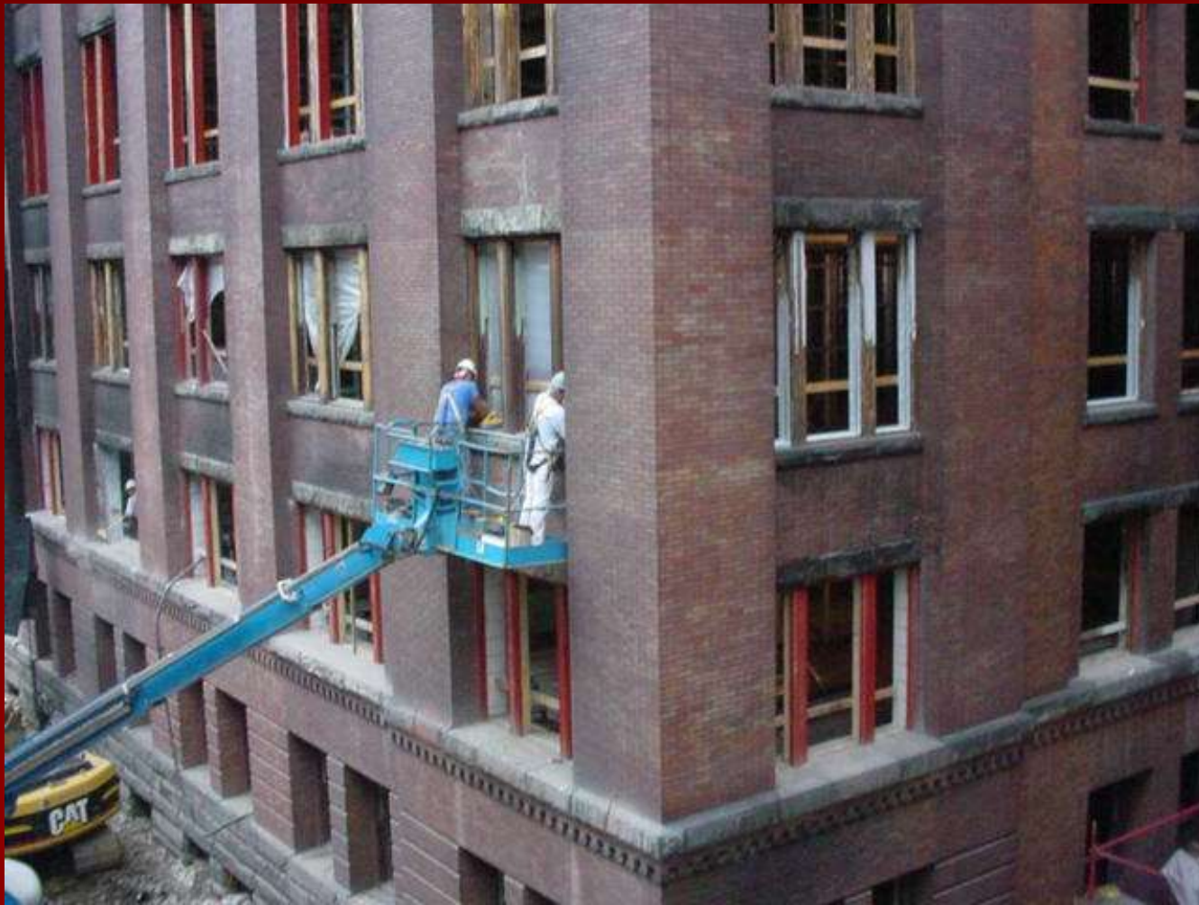
FIELD STRIPPING OF FRAMES
