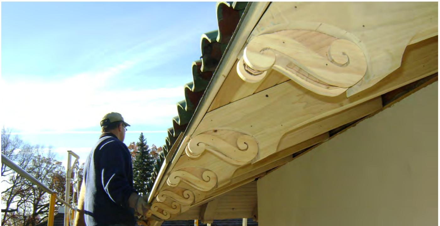
ABOVE: Nate's grandpa working on installing his recreated rafter tails and gutters. BELOW LEFT: Nate helping with stucco repairs. BELOW RIGHT: Updated photo of the house with a new roof, gutters and stucco work.
