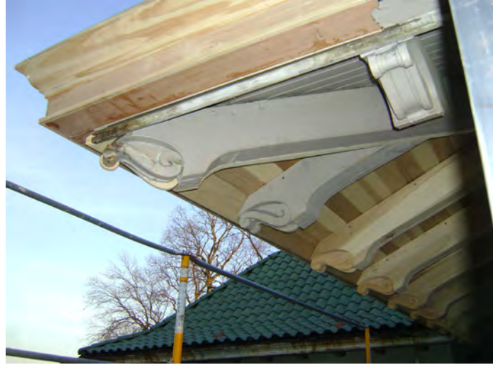
ABOVE: Nate's grandpa recreated the rafter tails from originals saved from the demolition as a pattern.
