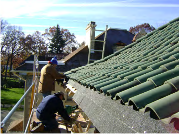
ABOVE: Roofers found salvaged green roof tiles to replace broken or damaged ones.
