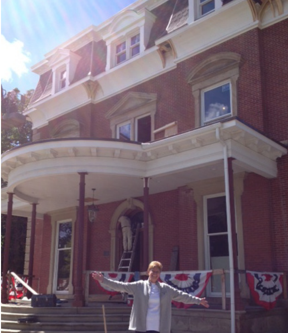
A visit to see the progress on the Steele Mansion in Painesville, Ohio, an Ohio historic tax credit project.
