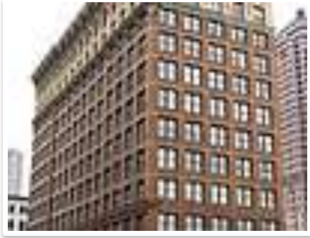
Columbus Savings and Trust Building
