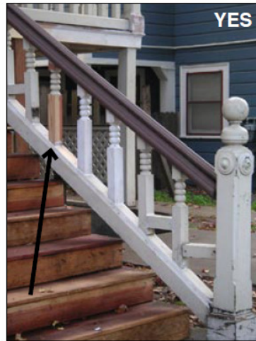
Guideline 1.4: It is appropriate to repair deteriorated building materials by patching, piecing-in, consolidating or otherwise reinforcing them. It is important to assess the cause of the damage and take steps to address the conditions that led to the deterioration.
