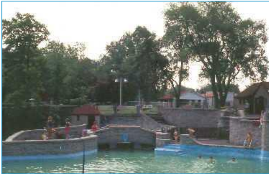
STRUCTURE – Columbus Grove Swimming Pool, Putnam County
