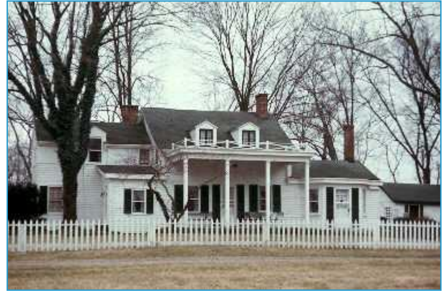
John Smith House, Hamilton County
