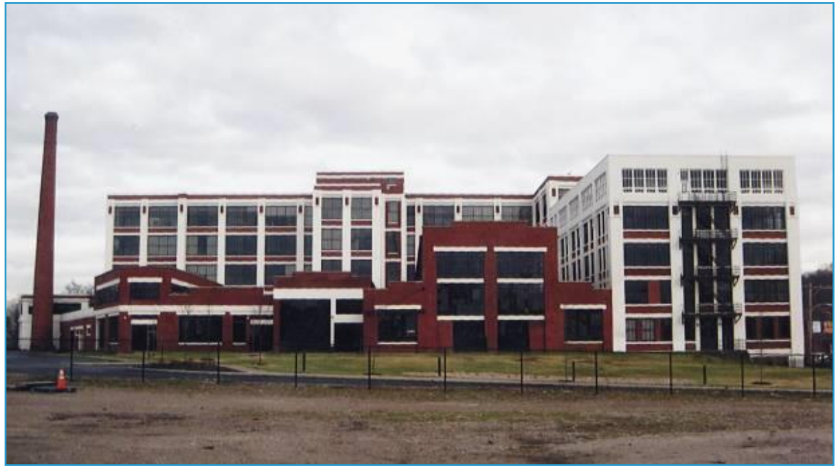
American Can Company, Hamilton County
