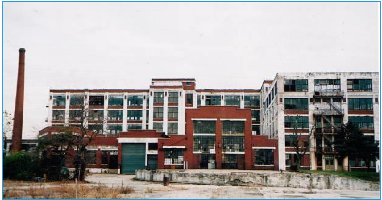
American Can Company, Hamilton County
