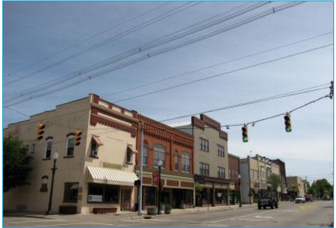
DISTRICT – Orrville Downtown Historic District, Wayne County
