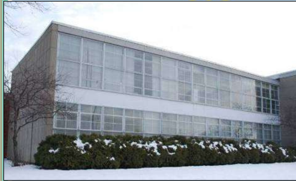
Horizontal ribbon window system
