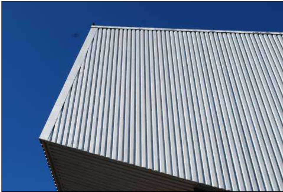
Vertical panel cladding
