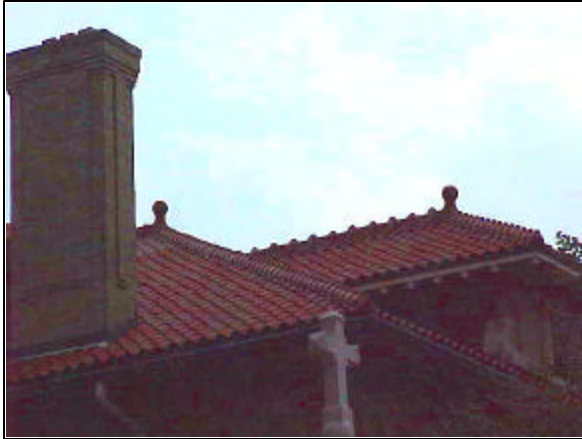
{Photo 18} Red tile roof with tile ridge cap
