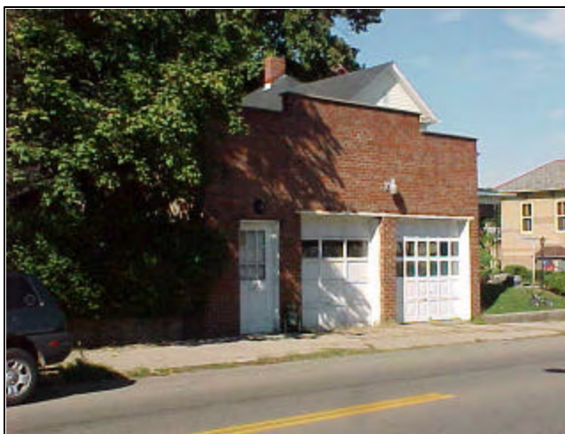
{Photo 62} Brick garage.
