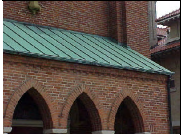
{Photo 19} Standing seam metal roof
