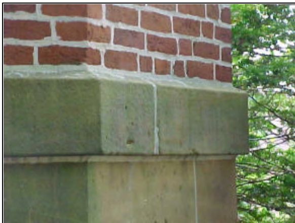
{Photo 1} Limestone water table between limestone foundation and brick wall.
