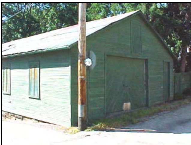
{Photo 63} Wood framed garage with original doors.
