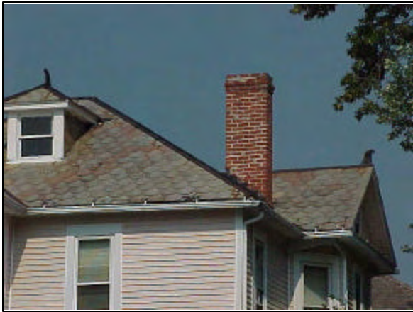
{Photo 20} Slate roof with ornamental metal ridge roll.
