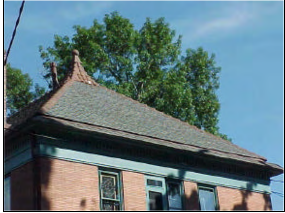
{Photo 21} Composite shingle with tile ridge cap
