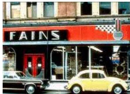
This 1930s Moderne storefront has gained significance over time and should be preserved. Photo: NPS files.
