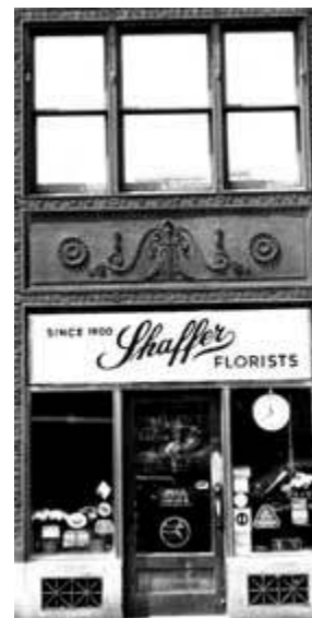
This finely detailed bronze storefront is typical of many constructed during the 1920s. The original grilles, spandrel panel and windows are all intact. Photo: NPS files.
