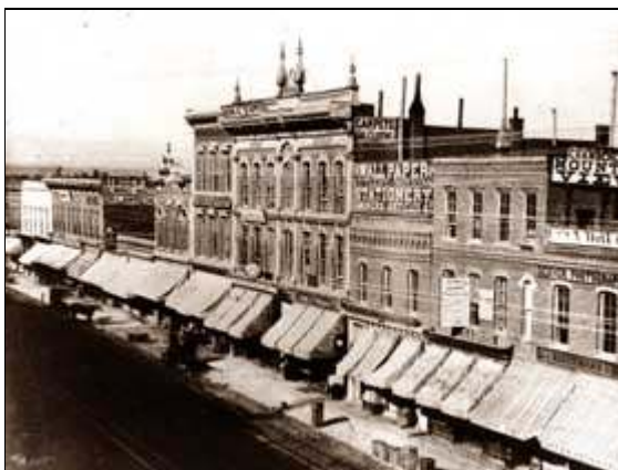
Try to locate old photographs or prints to determine what alterations have been made to the storefront and when they were undertaken. Awnings were common elements of storefronts at the turn of the century. Photo: NPS files.
