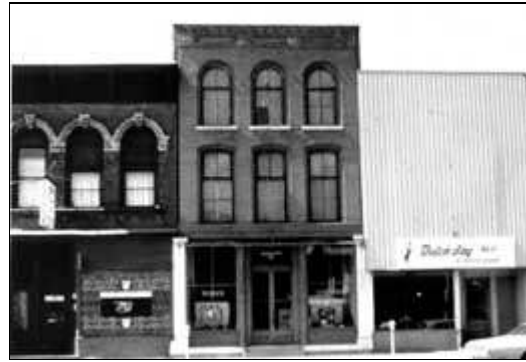
This photograph shows the impact of preserving historic storefronts. The one on the right has been totally obscured by a "modern" front added in the 1950s. Photo: NPS files.
