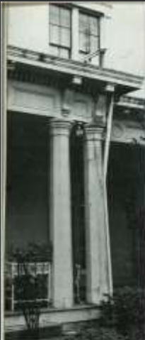
The roof drainage system has been neglected for such a long time that, as a result, the wood cornice and a fascia column are both severely deteriorated.
