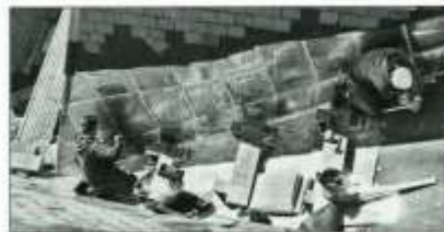
New copper valley flashing is installed as part of overall repairs to the historic slate roof and its drainage system.
