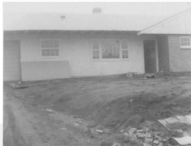
162 Cushwa Drive under construction. Photo courtesy of the Bombeck family.
