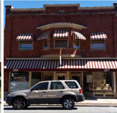
This was the first complete project with the Façade Enhancement Program. It is 205-207 S Washington Street. This project was approved for tuck-pointing, painting, window and door repair and roofing and resulted in over $16,000 in renovations.
