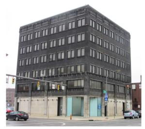
This view from 2018 shows the building stripped of its non-historic exterior alterations, allowing historic details to begin to emerge, including stonework at the first and second levels, and traces of a bracketed stone cornice along the roofline.
