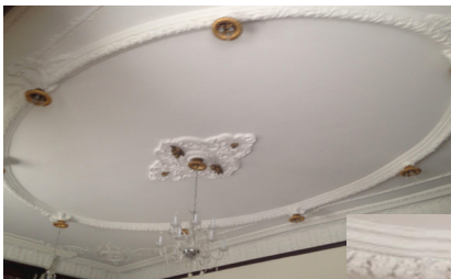
Left: Reception room ceiling and crown molding after restoration
