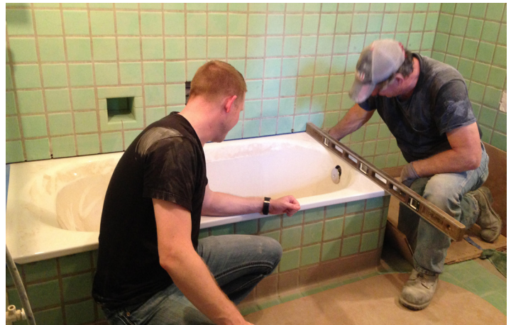
Above: Rookwood bathroom; a new tub was installed while maintaining the original tub surround
