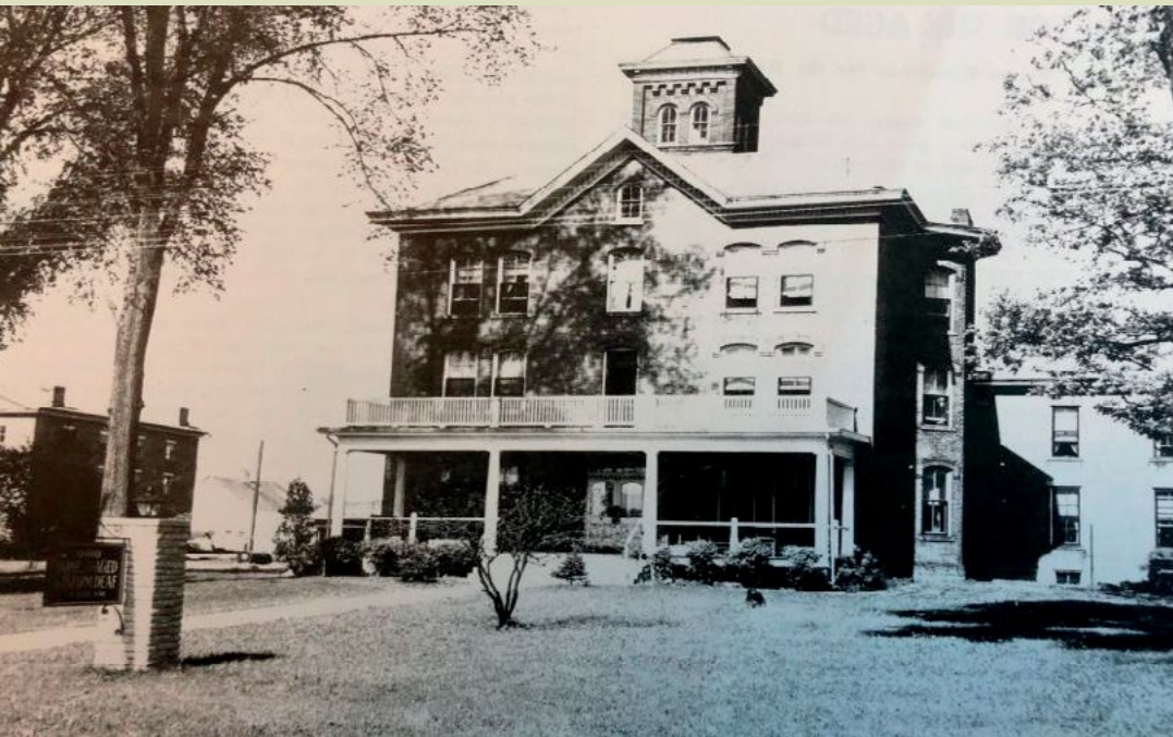
This is the original building purchased with the property named "Fairchild Building".
