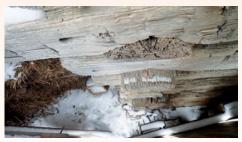
this barn had been replaced with concrete masonry unit (CMU) walls. Periodic tuck-pointing of the mortar between the stone will maintain the stability of the foundations and prevent their replacement.
