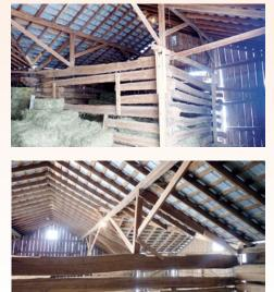
The logs used to construct the barns were typically sourced locally from the property. The wood was then hand hewn, meaning they have been flattened and squared using hand held tools. Because the process is performed by hand, the finished edges of the wood is often rough and choppy. This roughness provides a "rustic" appearance that is cherished today.
