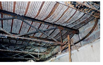
Modern steel joists are manufactured to meet standards in the building codes and will have small metal tags wired to their web members that will indicate the joist type and manufacturer. This information can be used to determine the maximum load the joist can support and can assist in designing modifications to strengthen the joists if needed. Many engineers are familiar with these joists and can provide details to strengthen them if needed.
