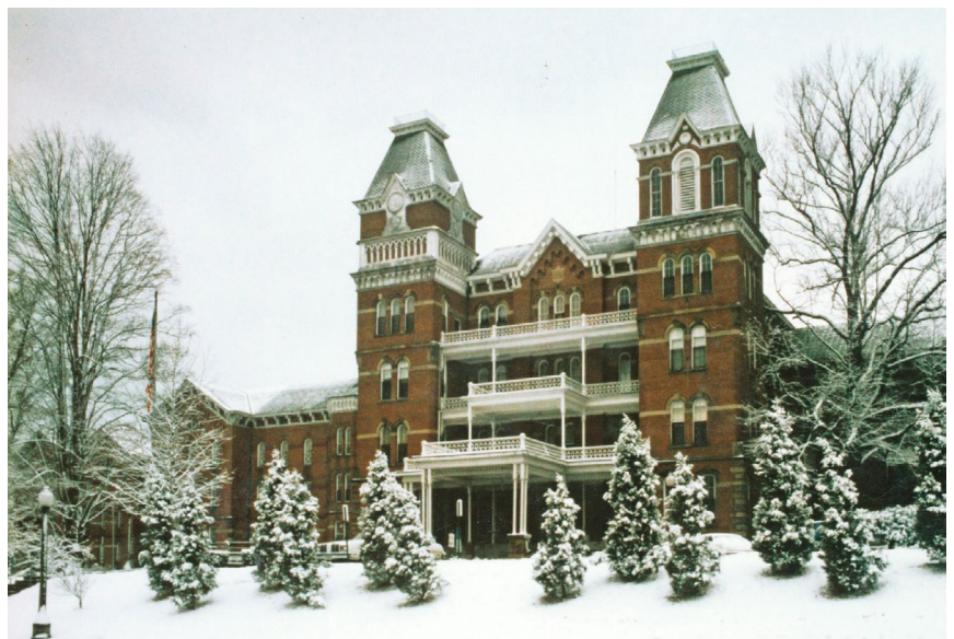
Athens Asylum, the largest building in Ohio at the time of its construction was the first of Levi Scofield's enormous legacy. He designed the Athens Asylum at age 26. Photo by: Tom O'Grady
